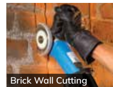
Brick Wall Cutting
