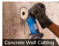
Concrete Wall Cutting
