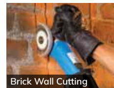
Brick Wall Cutting
